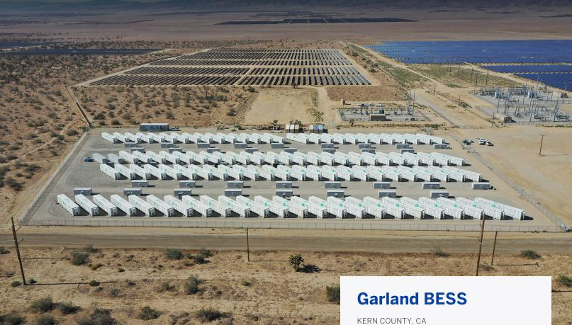
Rosendin Renewable Energy Group was contracted by Recurrent Energy to design and build the \$15 million battery energy storage system (BESS) in Kern County, California. The 88MW/352MWh Garland BESS project was added to the pre-existing 200 MW Garland Solar facility. Garland BESS used Powin batteries to provide four hours of battery storage to the grid, enhancing resource capacity by conserving clean, solar energy to be used during peak demand.
