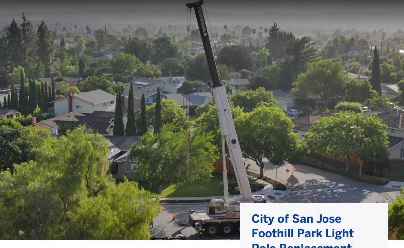
Rosendin replaced 3 – 800lb concrete light poles at Foothill Park for the City of San Jose. The existing poles were approximately 40-50 years old and were inaccessible for servicing due to the steep terrain. A crane was used to reach 250' from the roadway to remove the old poles and replace with new hinged poles with internal winches for future servicing. The new LED fixtures will make the park brighter and safer for years to come.
